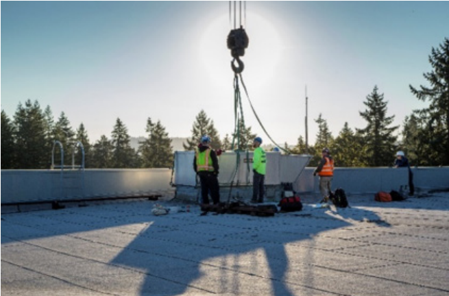
PREPARING EXISTING UNIT FOR REMOVAL
