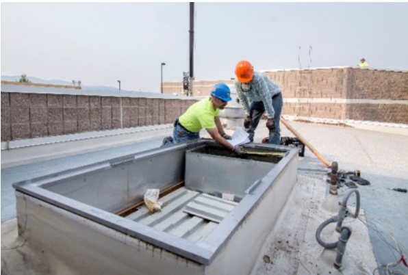
UTILIZING EXISTING ROOF CURB WITH CURB ADAPTER
