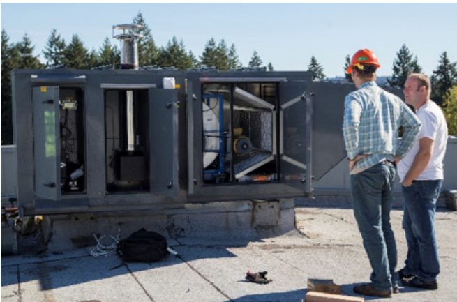
NEW UNIT INSTALLATION
