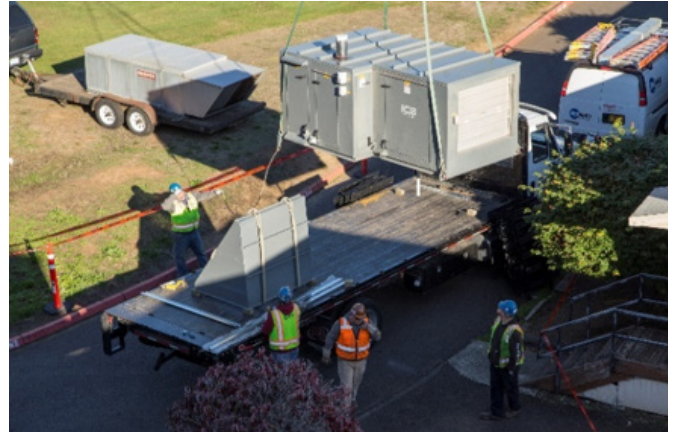
REPLACEMENT C-RTU CRANE PICK
