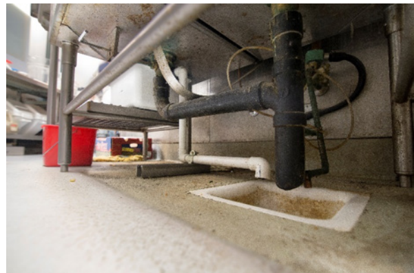
CONDENSATE DRAIN TERMINATION
