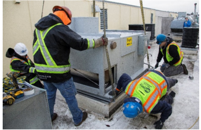
REPLACEMENT C-RTU PLACEMENT
