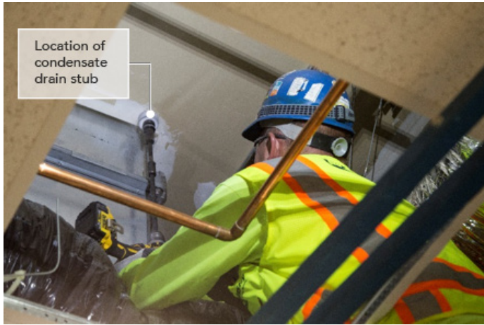
CONDENSATE DRAIN PENETRATION (CEILING OR BOTTOM VIEW)
