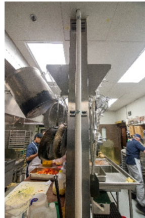
DRAIN ENTERING KITCHEN
