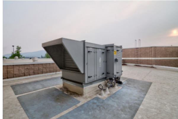
C-RTU INSTALLED
