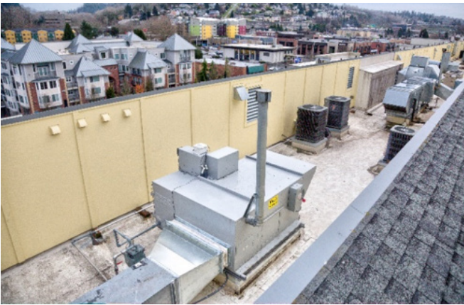
NEW C-RTU INSTALLED
