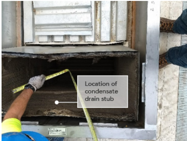
SUPPLY DUCT OPENING (ROOF OR TOP VIEW)
