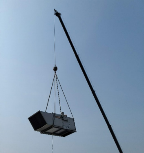
EXISTING UNIT BEING REMOVED
