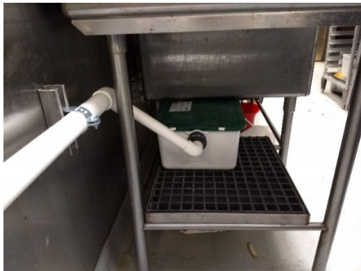
CONDENSATE NEUTRALIZER TANK
