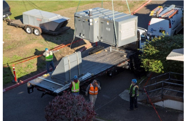
REPLACEMENT C-RTU CRANE PICK
