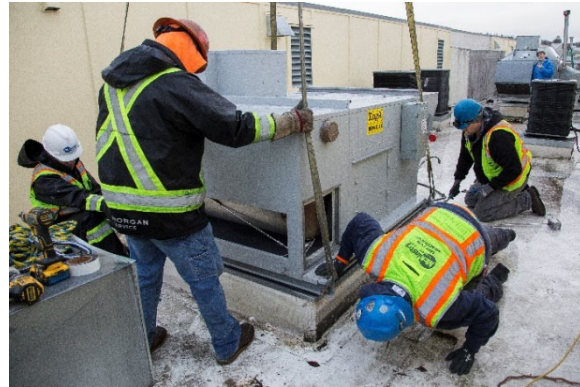
REPLACEMENT C-RTU PLACEMENT
