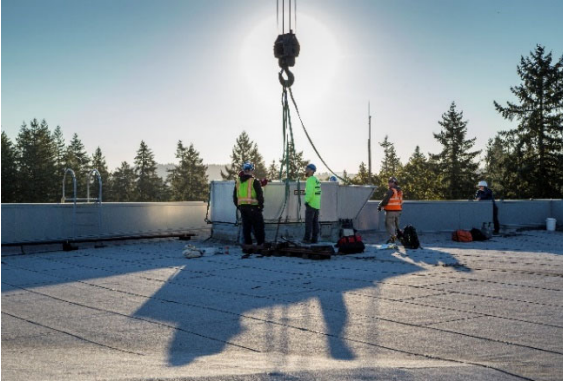
PREPARING EXISTING UNIT FOR REMOVAL
