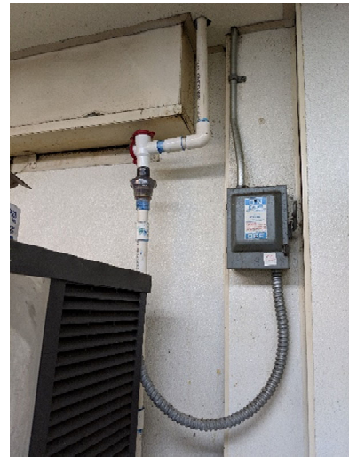
CONDENSATE LINE IN KITCHEN WITH WINDOW FOR VERIFYING CONDENSATE FLOW
