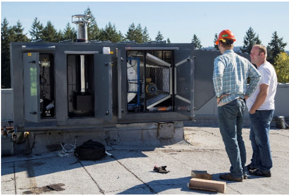
NEW UNIT INSTALLATION
