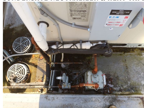
CONDENSATE NEUTRALIZER & HEAT TAPE
