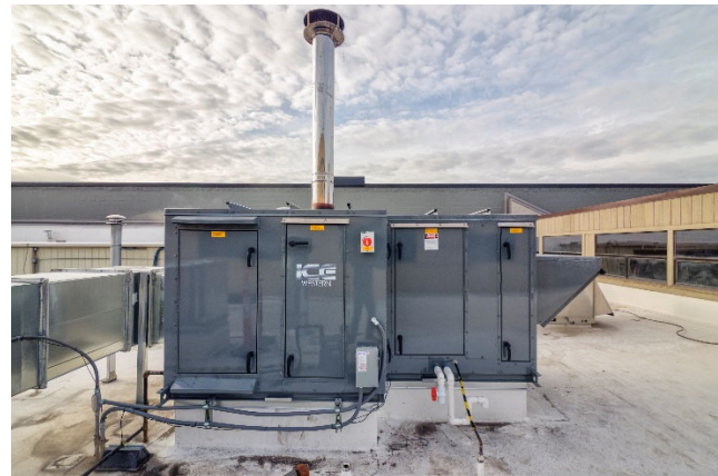
C-RTU INSTALLED
