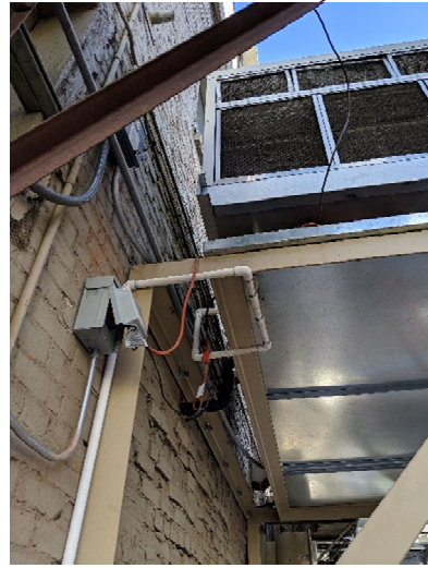
CONDENSATE LINE IN KITCHEN WITH WINDOW FOR VERIFYING CONDENSATE FLOW
