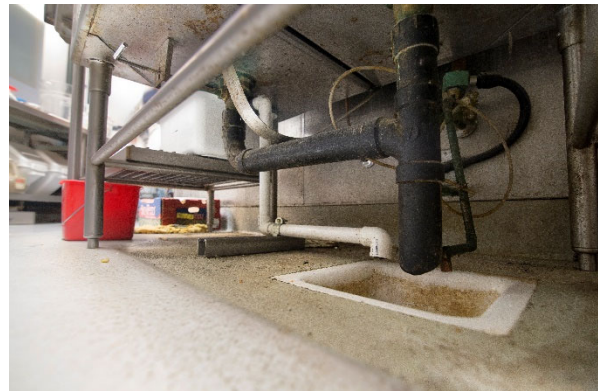
CONDENSATE DRAIN TERMINATION
