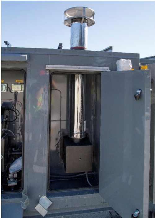
FIGURE 26 – FLUE BEFORE EXTENSION INSTALLED
