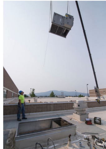
REPLACEMENT C-RTU CRANE PICK
