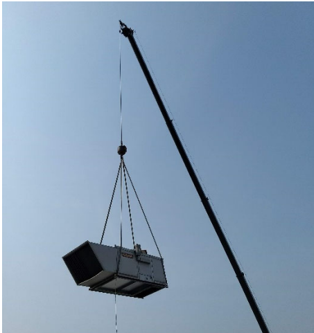
EXISTING UNIT BEING REMOVED
