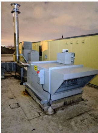
NEW C-RTU INSTALLED
