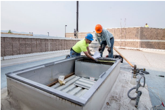
UTILIZING EXISTING ROOF CURB WITH CURB ADAPTER
