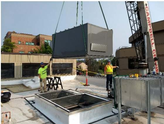
C-RTU CRANE PICK
